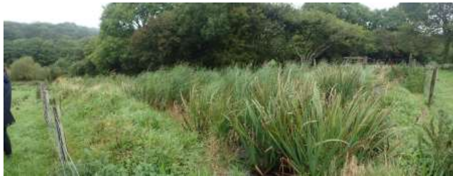
The reedbed filter cleans the water before it returns to the river
