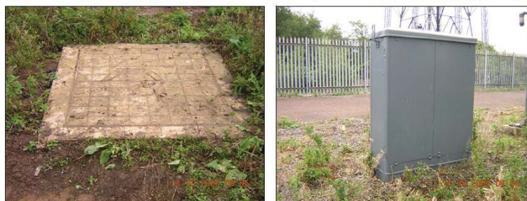
Typical cross-bonding arrangements involve either a buried pit with a manhole or an above ground pillar
