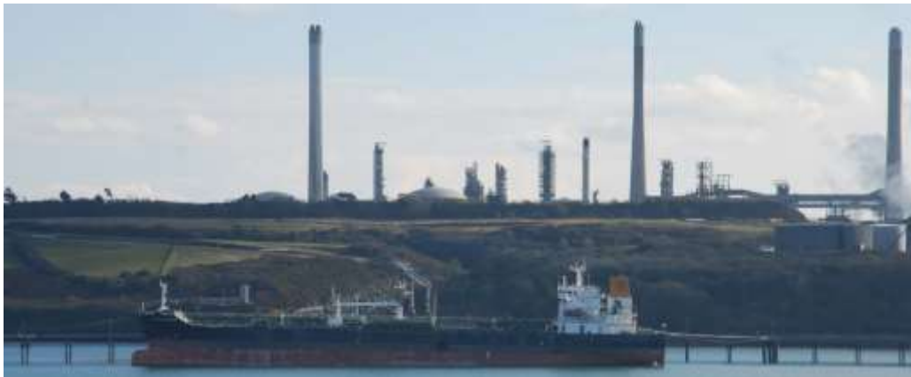
Milford Haven- refinery
