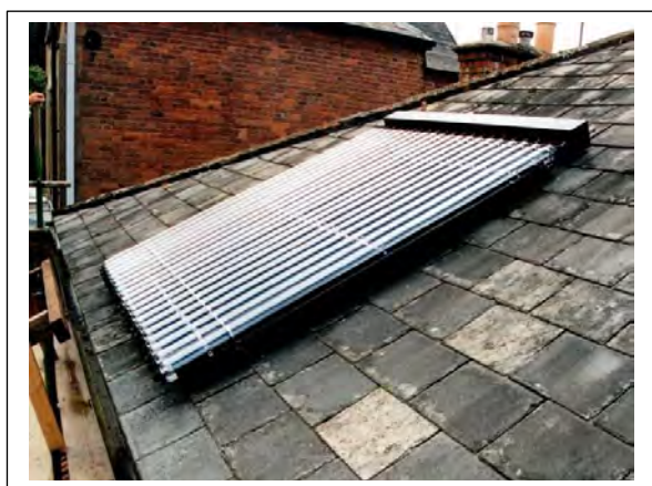
Solar hot water panel (evacuated tube system)
