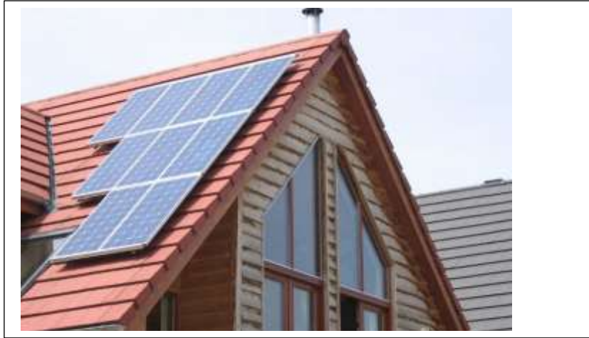
Retrofit solar PV panel
