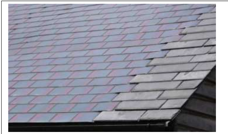
Retrofit solar PV panel
