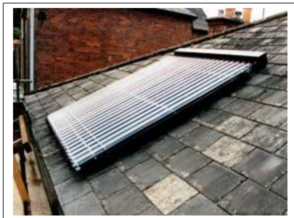
Solar hot water panel (evacuated tube system)
