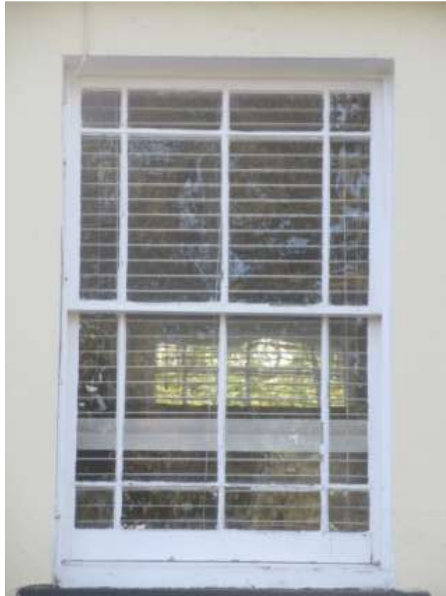
Figure 18 - Victorian marginally-glazed sash window
