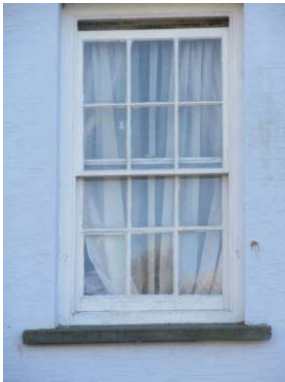
Figure 17 - early 19th century small-paned sash window
