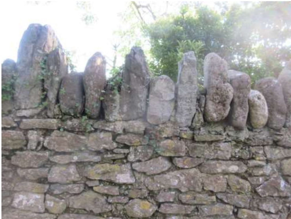
Figure 5 - various types of wall copings
