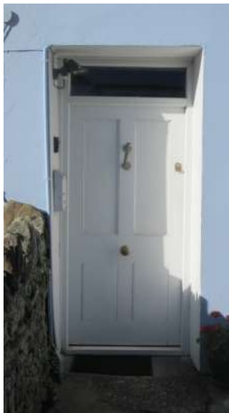
Figure 23 - typical Victorian four-panel design
