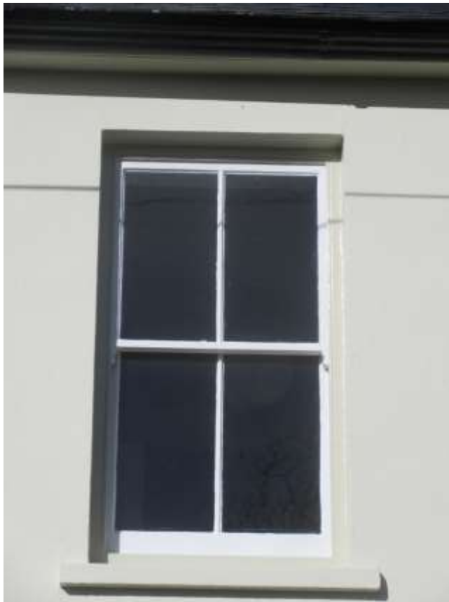
Figure 19 - Victorian four-paned window
