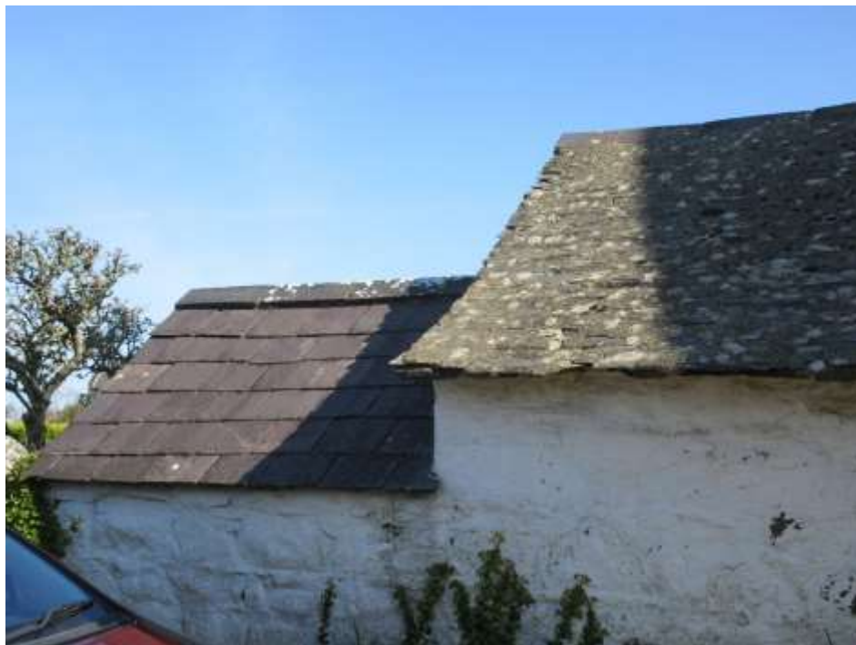
Figure 58 - local 'slurried' slate and North Wales slate
