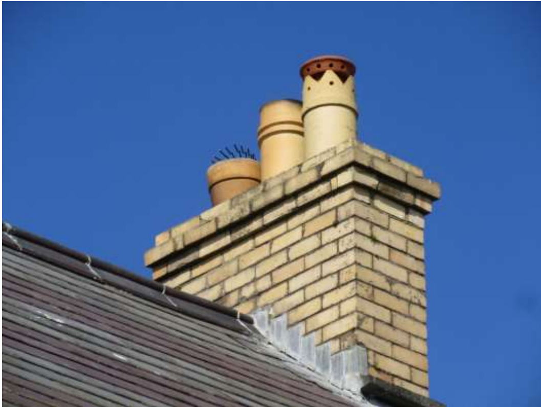
Figure 61 - stack built of buff Flintshire brick
