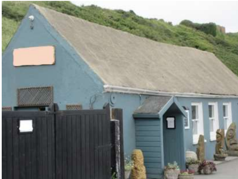
Figure 20 - grouted roof
