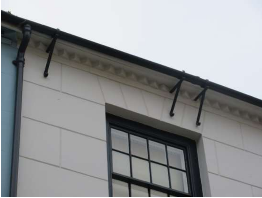
Figure 50 - 'cogged' eaves detail
