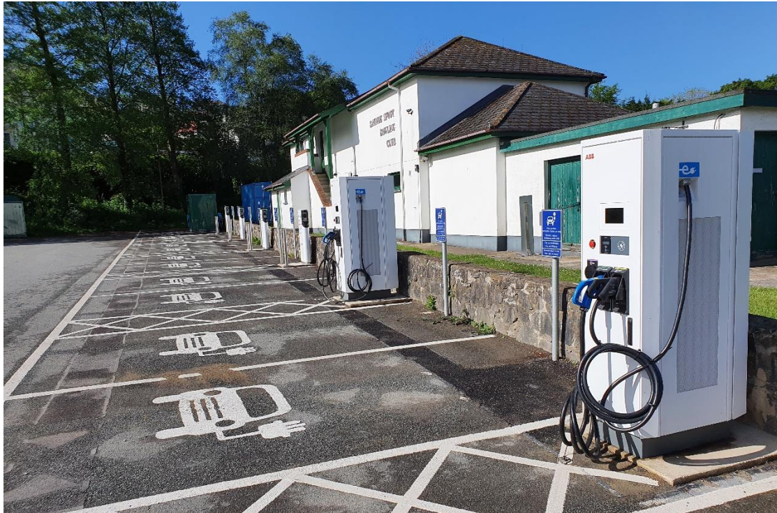
Example of Electric Vehicle Charging Points Installed
