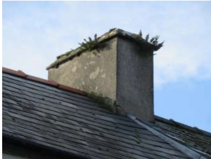
Figure 20 - typical rendered chimney stack
