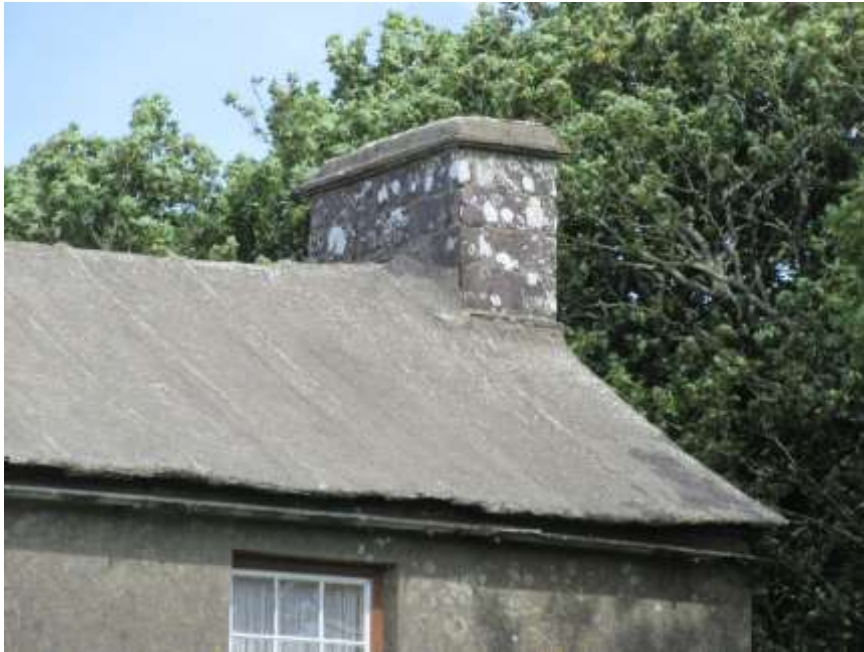
Figure 20 - 'grouted' roof
