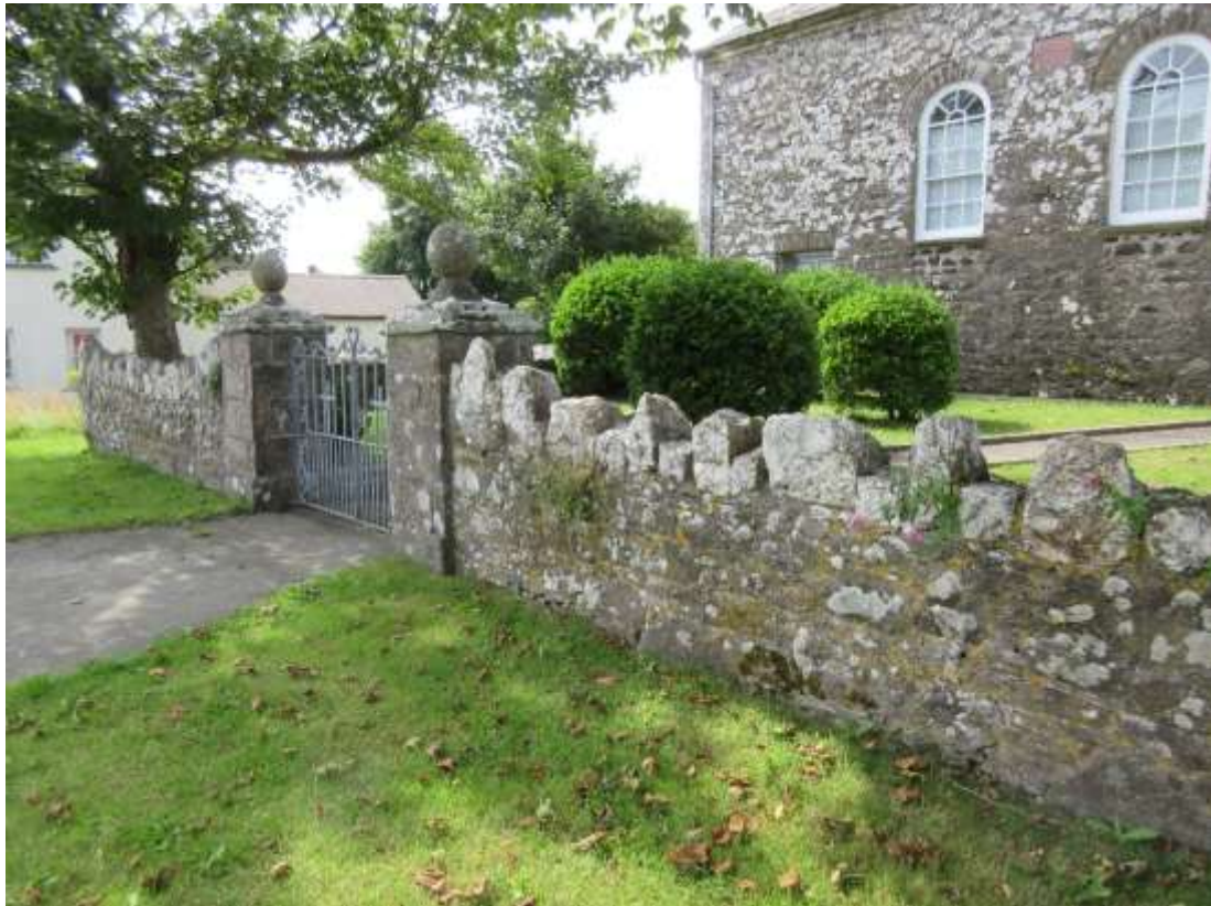
Figure 13 - chapel boundary walls with quartzite copings
