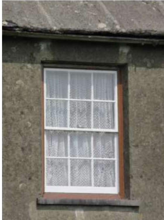
Figure 15 - 12-paned sash
