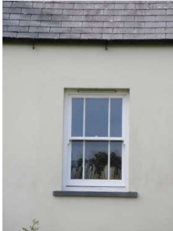
Figure 16 - marginal-paned sash
