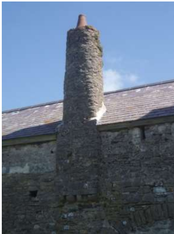
Figure 16 - C16 round chimney, Caldey Priory
