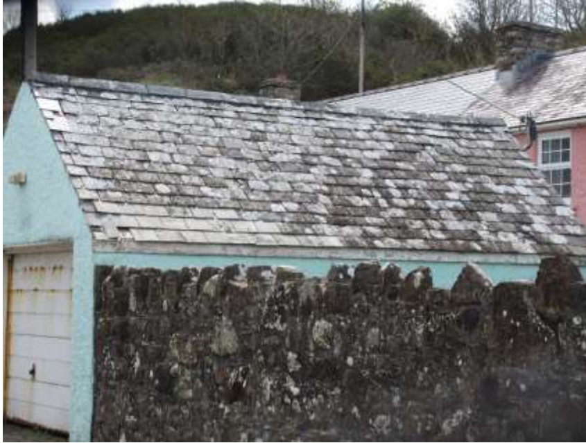
Figure 24 - roof using local slates
