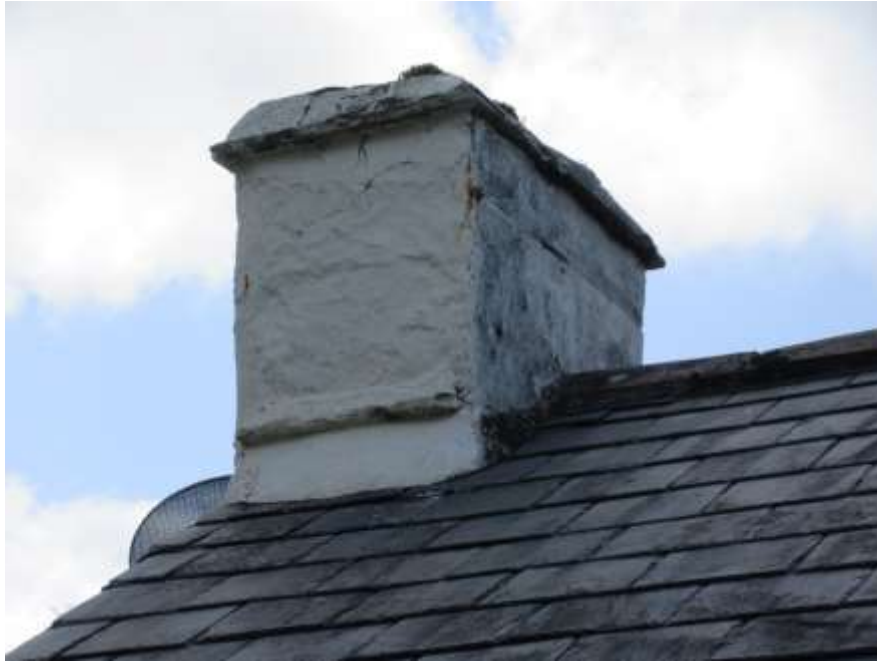
Figure 28 - stone chimney stack, Grove Place
