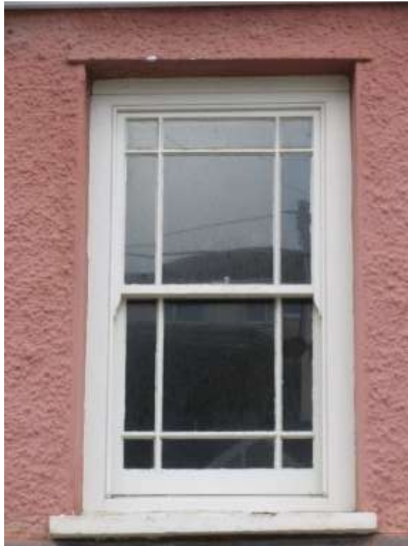
Figure 20 - marginal-paned sash
