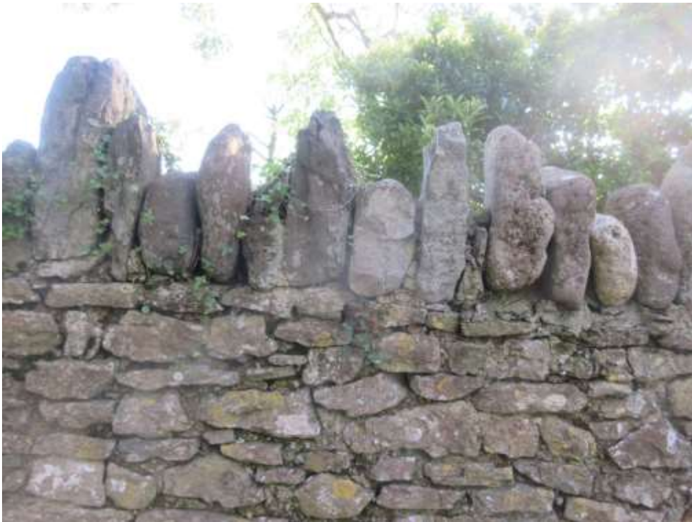
Figure 5 - various types of wall copings
