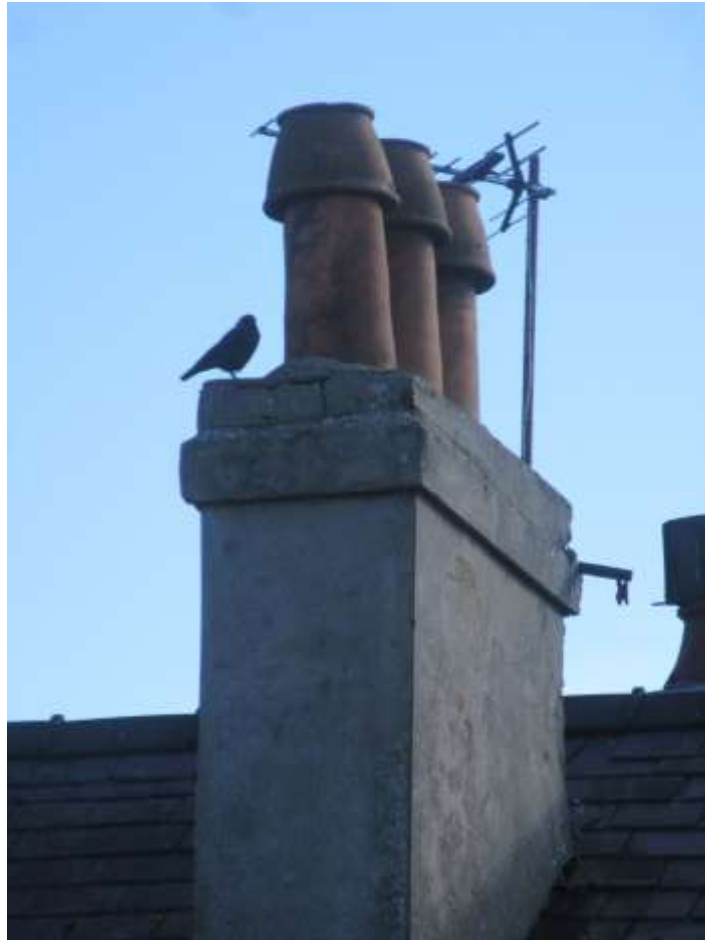
Figure 30 - rendered chimney with unusual pots
