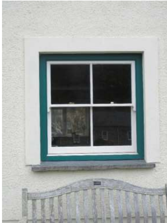
Figure 18 - 4-paned sash window
