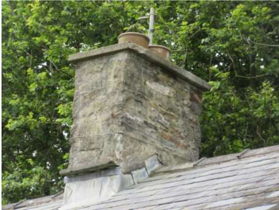
Figure 22 - stone chimney stack
