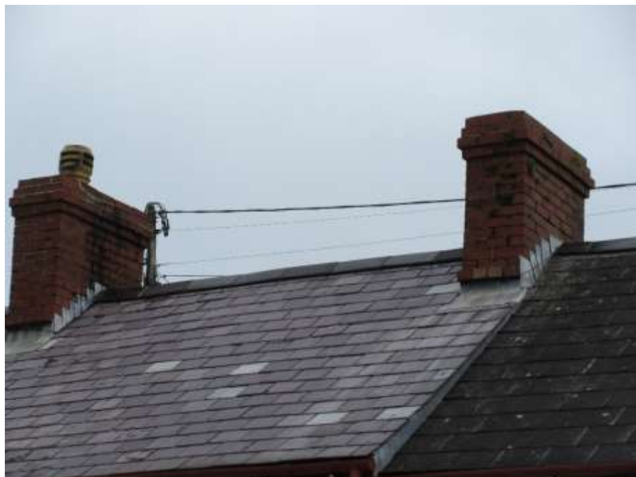
Figure 23 - chimneys of Porthgain brick
