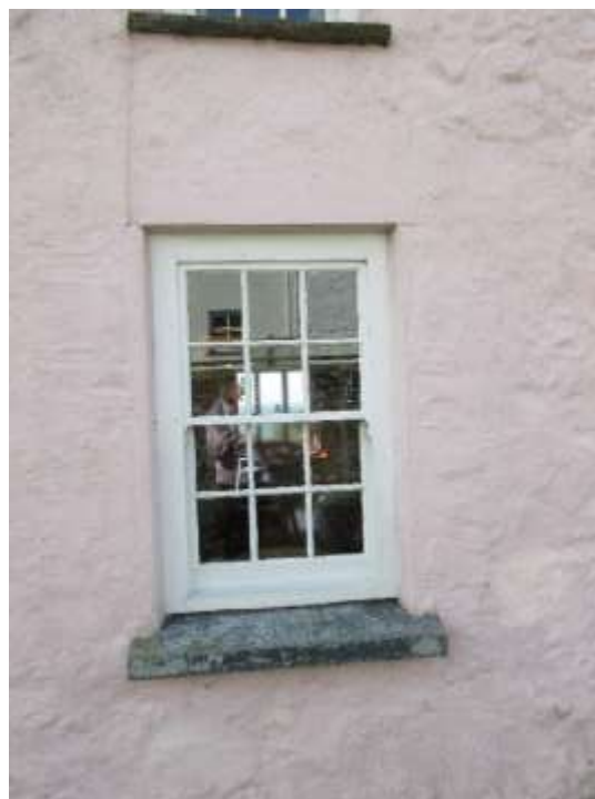
Figure 29 - 12-paned sash window
