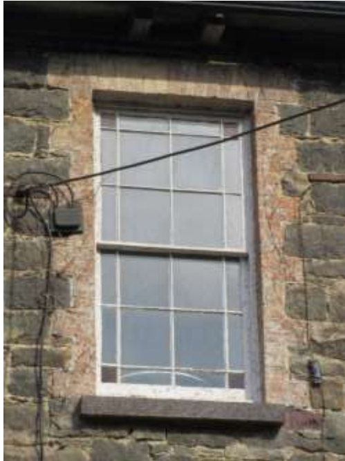
Figure 30 - marginal-paned sash window
