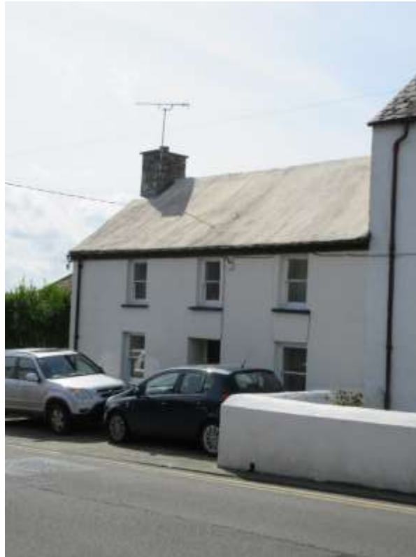
Figure 34 - grouted roof
