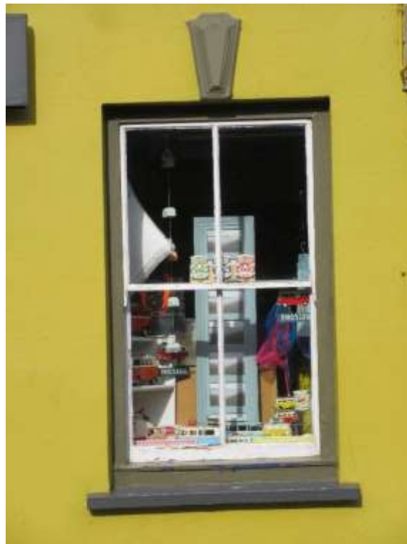
Figure 31- four-paned sash window
