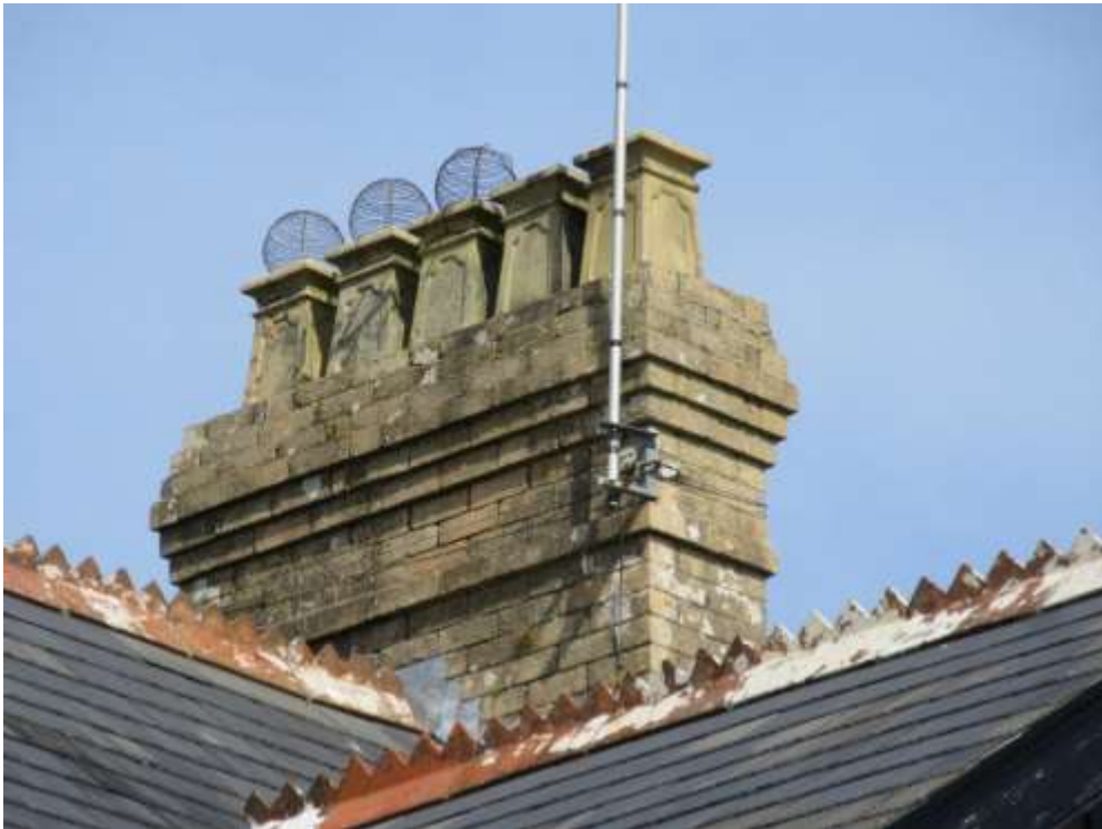
Figure 37 - yellow brick chimney stack
