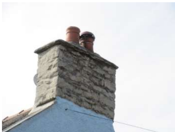
Figure 35 - stone chimney stack
