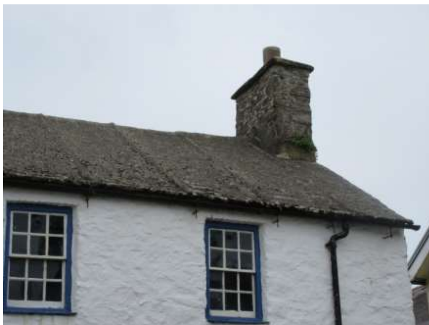
Figure 45 - cement grouted roof
