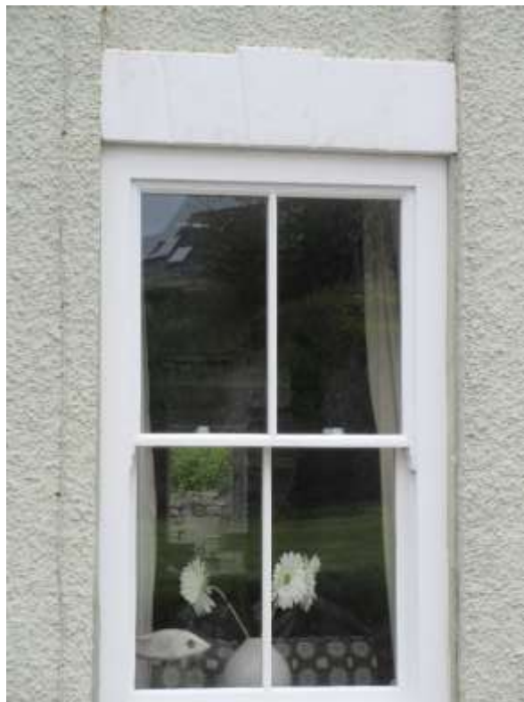
Figure 41 - Later C19 4-paned sash window
