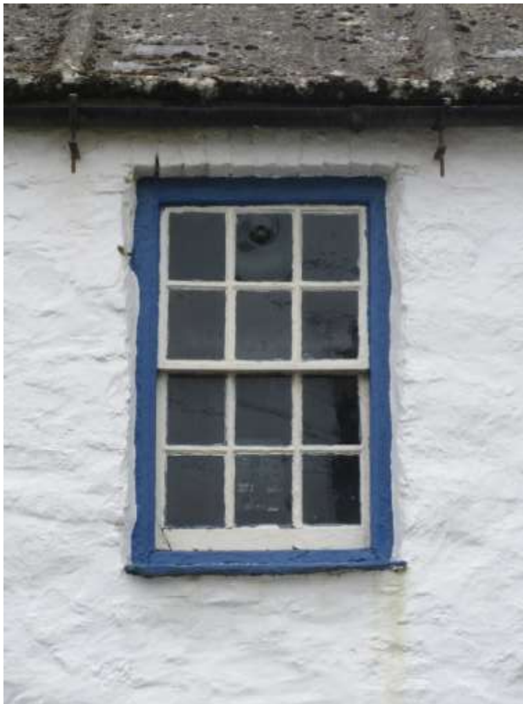
Figure 39 - Early C19 12-paned sash window
