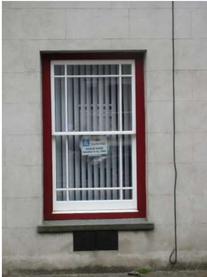
Figure 40 - Later C19 marginal-paned sash window
