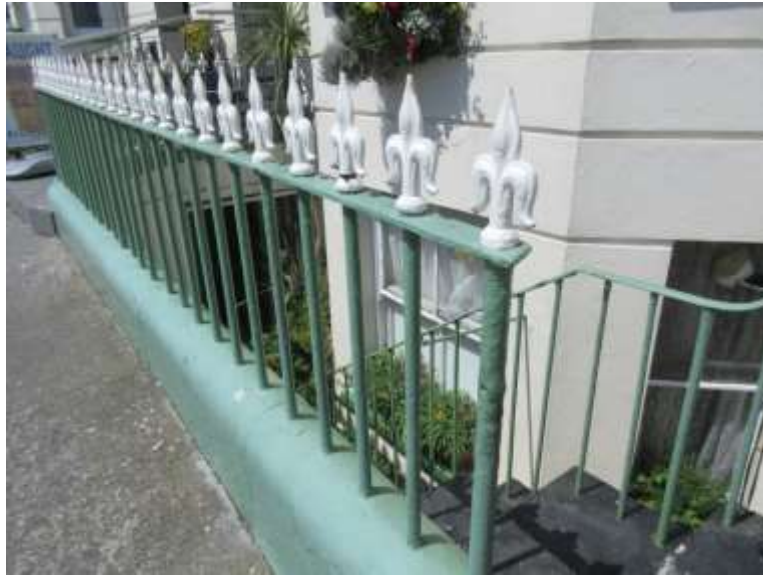
Figure 60 - locally-made cast iron Victorian railings
