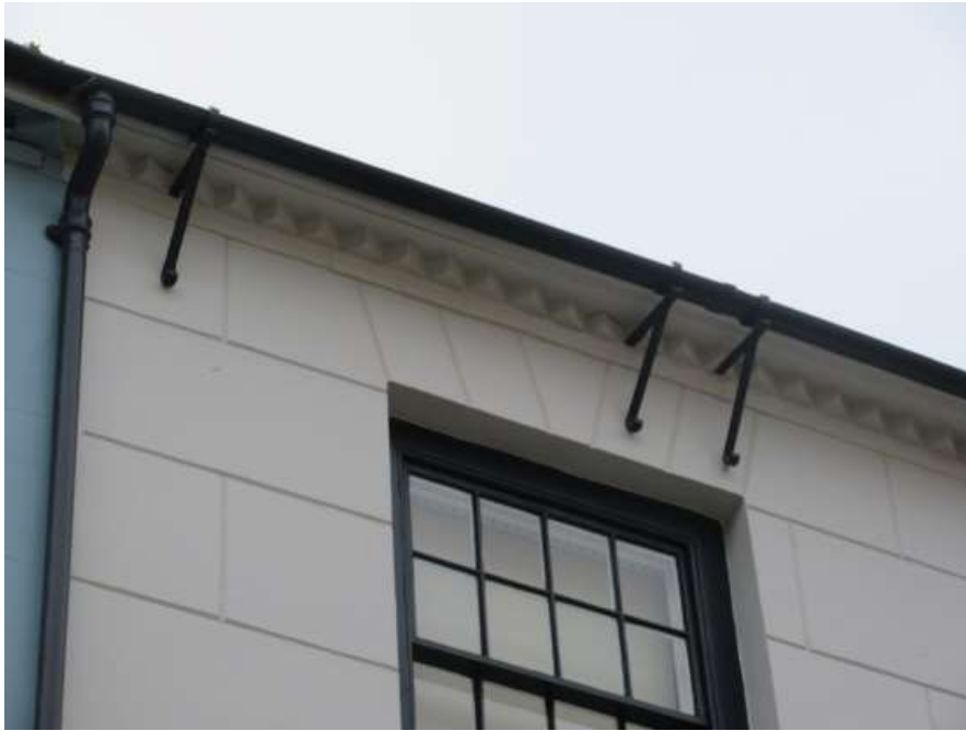
Figure 50 - 'cogged' eaves detail
