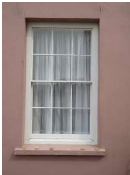
Figure 40 - typical 12-paned early C19 sash window with elegant glazing bars
