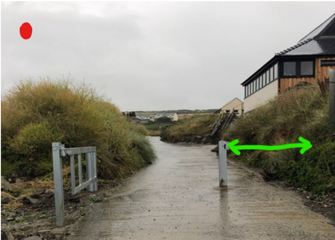
'Installed barrier on northern slipway in its open configuration (viewed from the beach looking inland) showing the permanently maintained opening indicated by the green arrow''.
