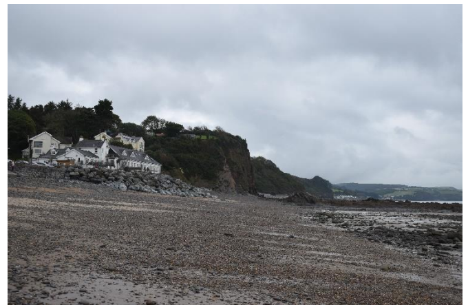
View north-east along coast from Wiseman's Bridge, showing mixed woodland and scrub along coastal cliffs.
