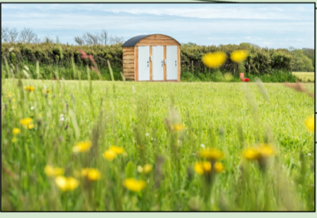
3 WC and Urinal Pod
