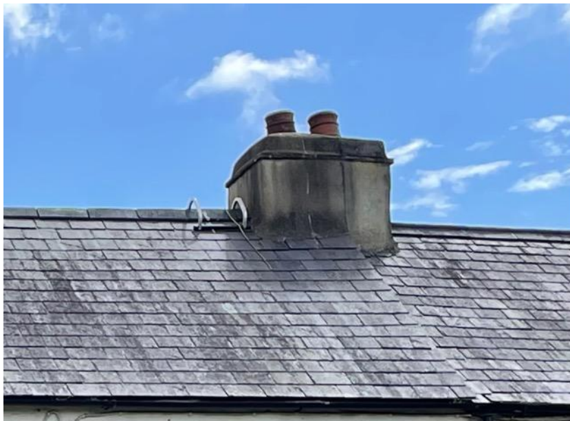
Figure 19: Photograph showing a smooth rendered chimney
