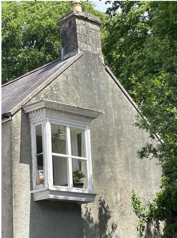
Figure 13: Photograph showing a cantilevered rectangular bay window
