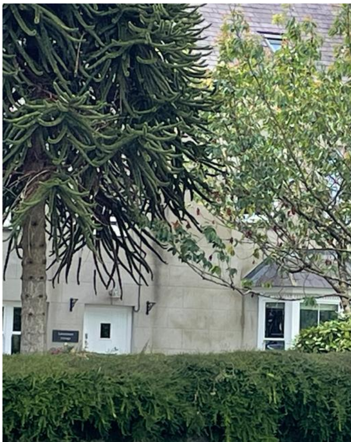
Figure 8: Photograph showing a building with scribed render
