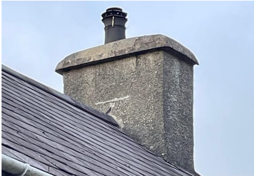
Figure 20: Photograph showing a roughcast rendered chimney.
