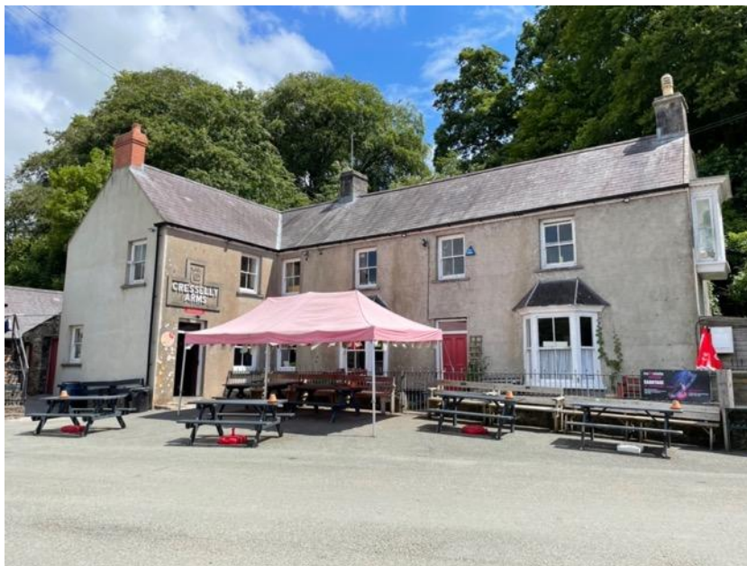
Figure 17: Photograph showing gabled and slated roof
