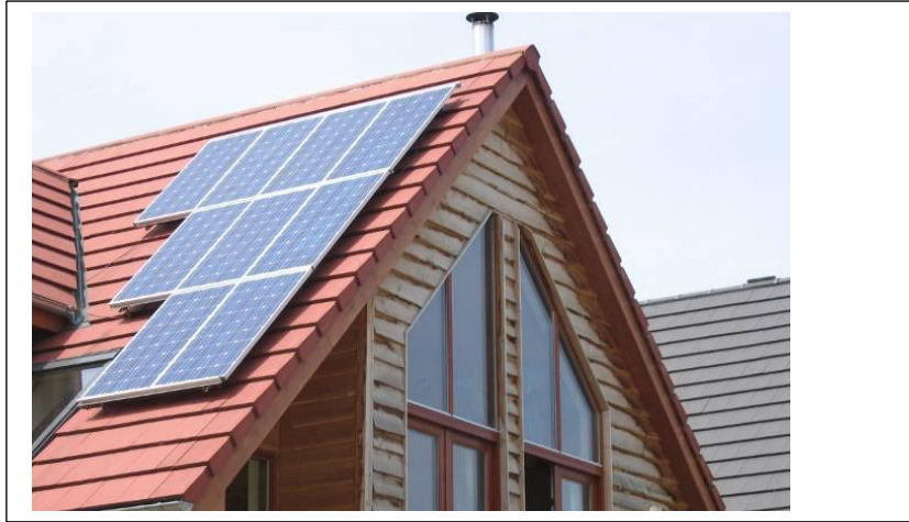
Retrofit solar PV panel
