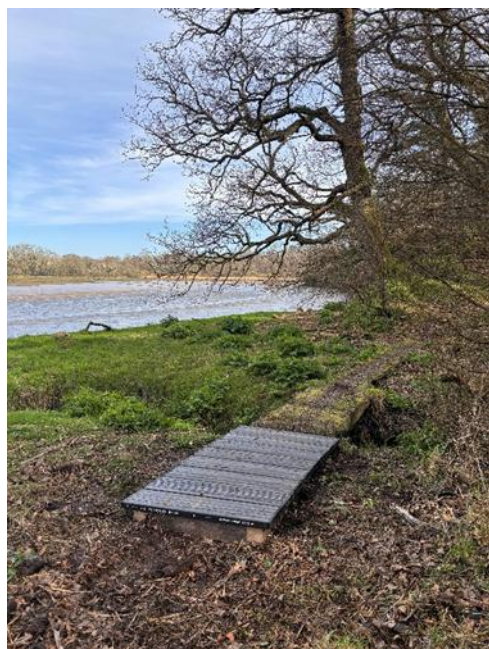
Boardwalk after repairs path 25/9
