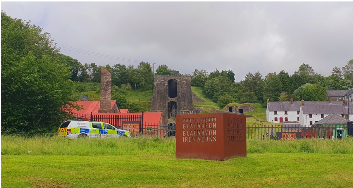
Historic Blaenavon Ironworks.
