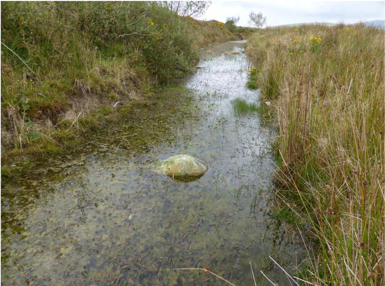
A wet ditch / flush system has been created, which collects spring inputs and surface drainage water from the upper central part of the site. Through shallow profiling and partially excavating along contour lines rather than down them, the flow is slowed and a drawdown zone with bare clay and developing flush vegetation has been created.
