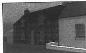
Image from south-west - Before
