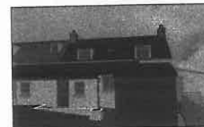
Image from north-west - Before
