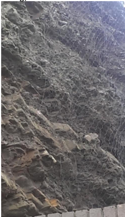
Appendix K - Previous measures to curtail outcrop degradation (mesh netting)
