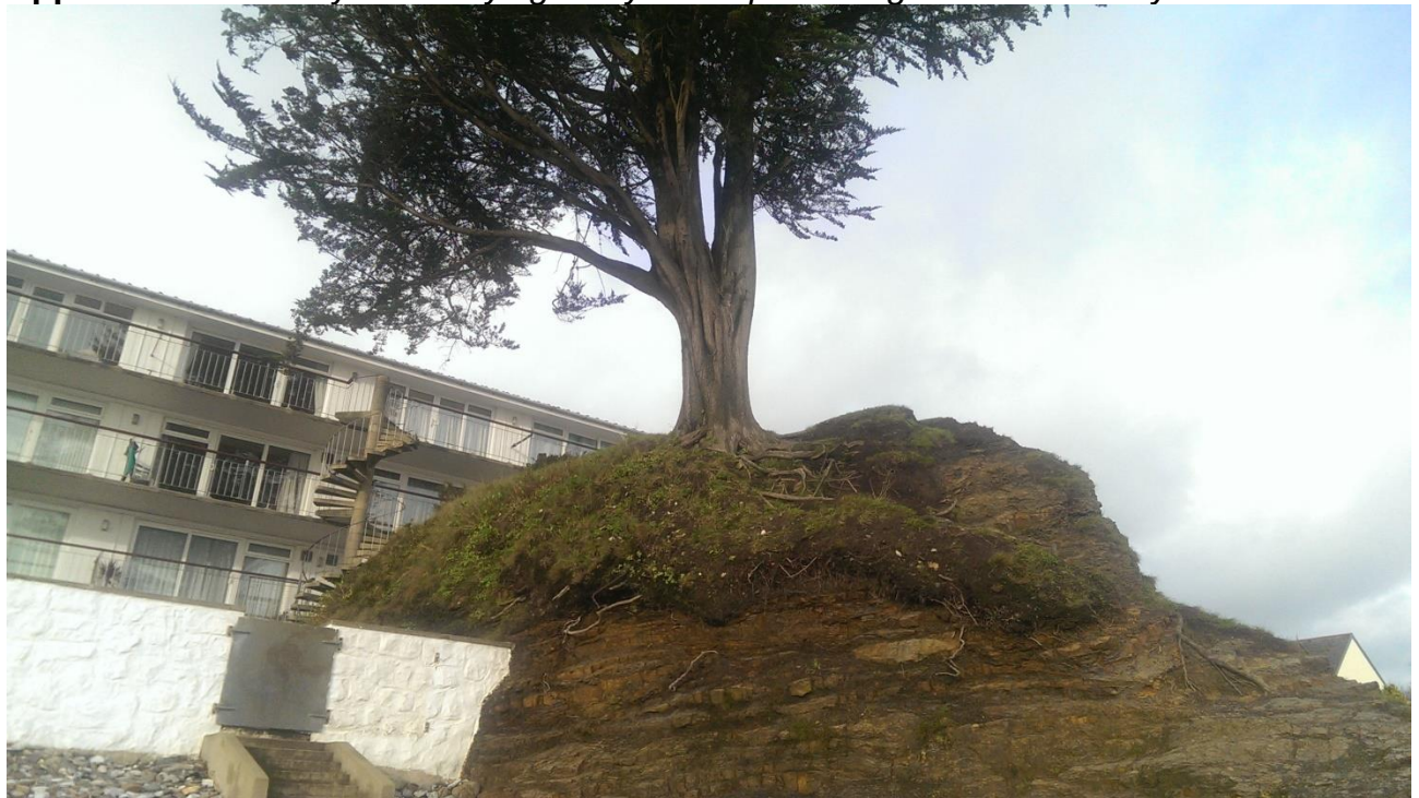
Appendix F – Soil layer overlaying rocky outcrop showing undercut soil layer
