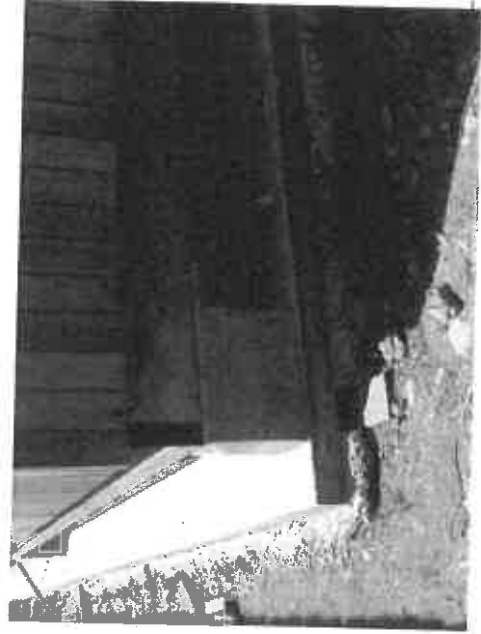
Photo 3: Reinforced Concrete Slab referred to (South-East corner)
