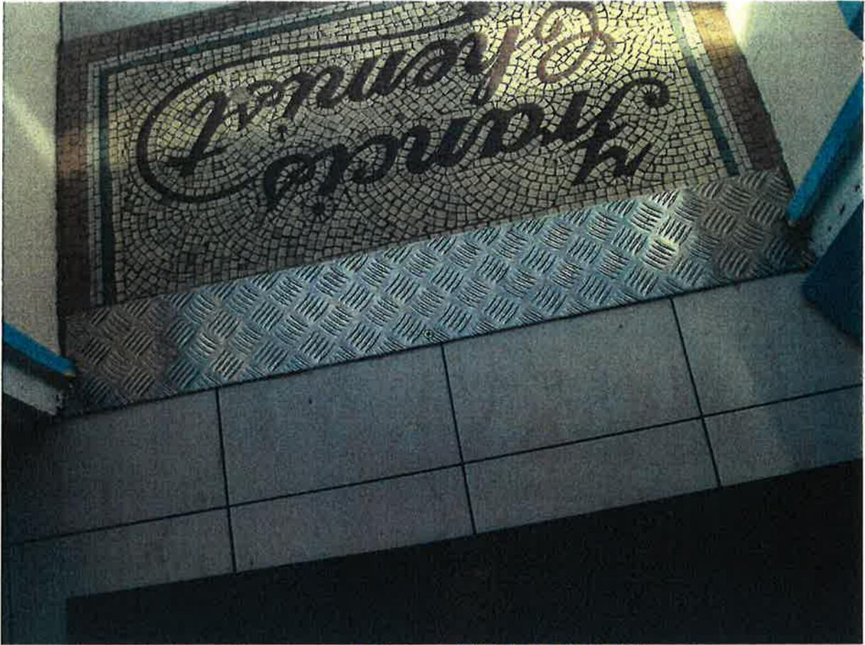
Photograph F – steel plate installed to threshold 2016
