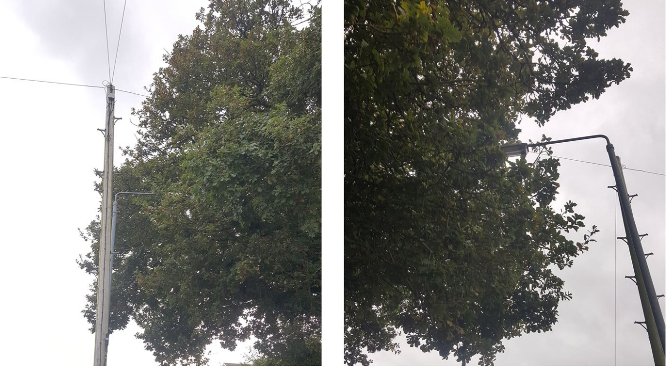
Image 8 – Foliage in proximity to Streetlight – Images taken from both sides of street light Telecommunications cables also visible
