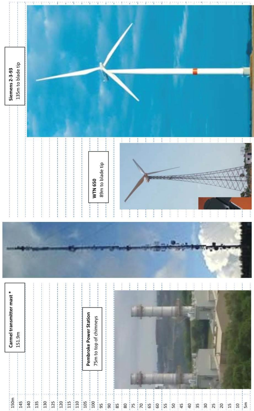
Figure 3: Turbine types and size comparison - medium large sized turbines
